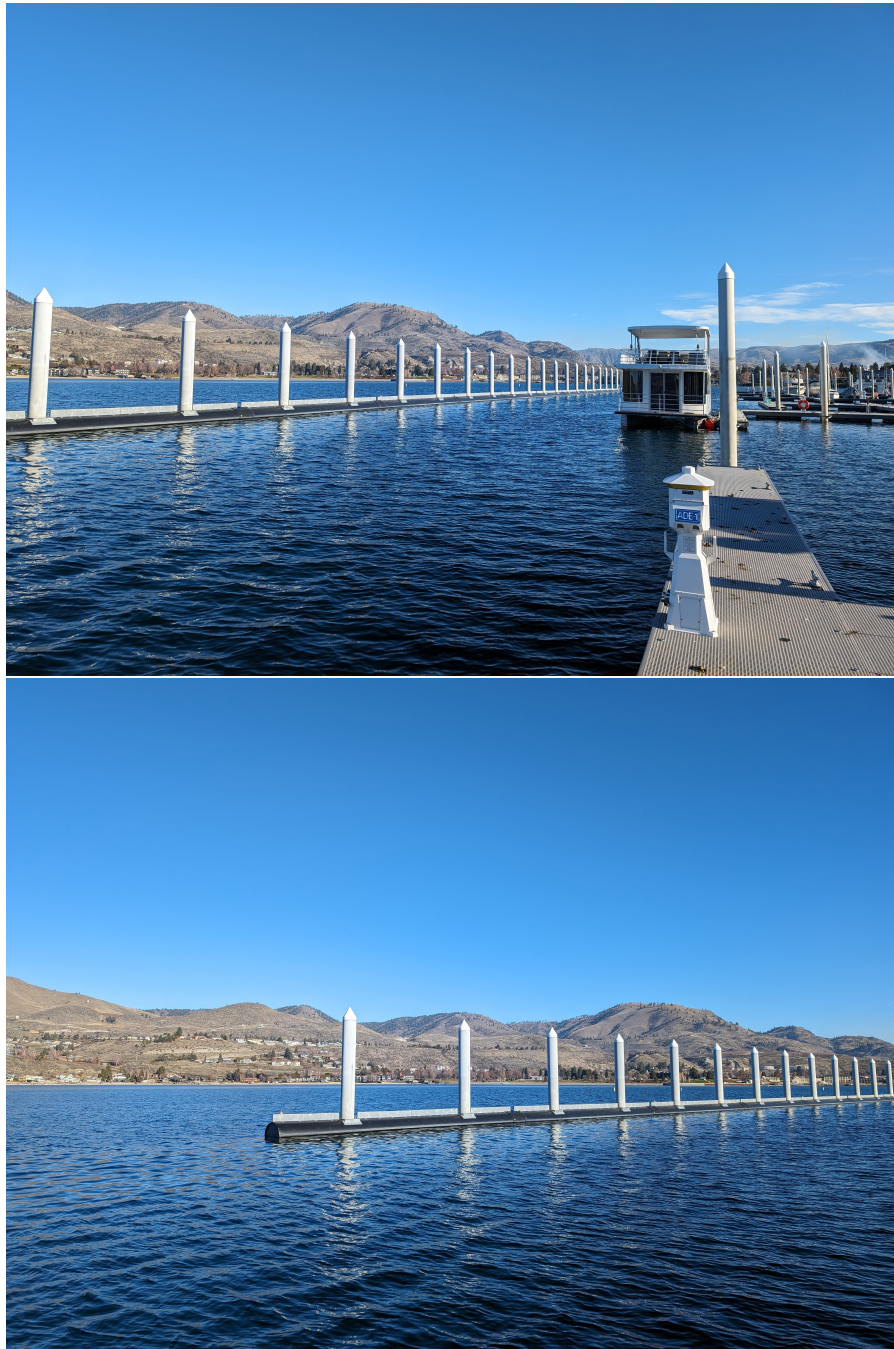
Figure 9: Sunset Marina (SUN) is a large, wave protected, private marina with floating docks. This area is perennially deep, with water depths up to 40 ft (12 m) at high pool.
